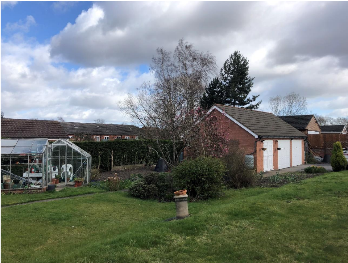
Existing garage from garden of 97 Boultham Park Road, boundary with no. 95 in background
